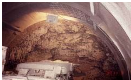
Obr. 6. Pohľad na čelbu a raziaci stroj AM-50 (Alpine) Fig. 6. View on the working face and embossing machine AM-50 (Alpine)
