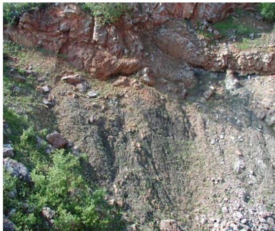
Fig. 17. General view on thrust plane at the level of the 10A storey.
