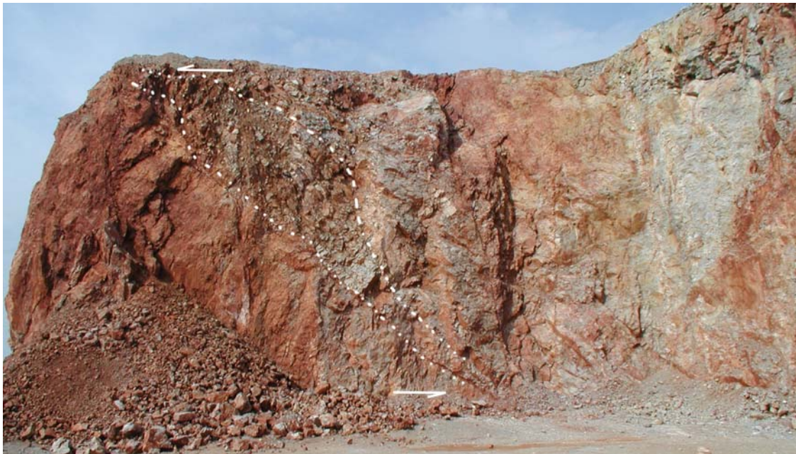
Fig. 9. Sigmoid course of foliation resulted from increased progressive deformation on the 7C storey.
