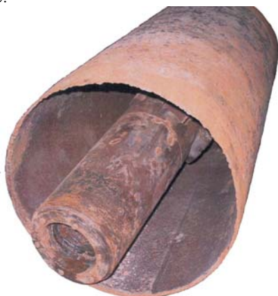
Fig. 2. A swivel in the protective pipe of leading head of the gas pipeline
