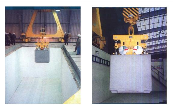
Fig. 3. Manipulation of the container during the process of its placing into the chamber of storage place.
