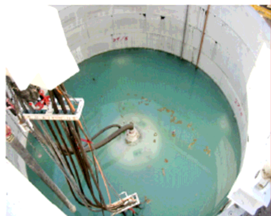
Fig. 4. Vertical drilling below the groundwater.
