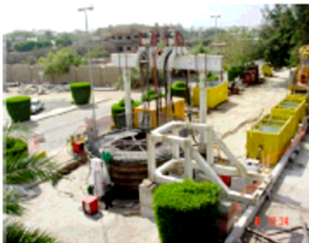
Fig. 11. Deployment of a shaft sinking unit in Jeddah Saudi Arabia.
