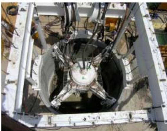
Fig. 3. Shaft boring unit gripped in the launch section.
