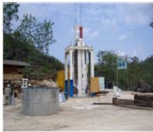
Fig. 6. Shaft sinking equipment VSM 2500 for a 100m deep shaft.
