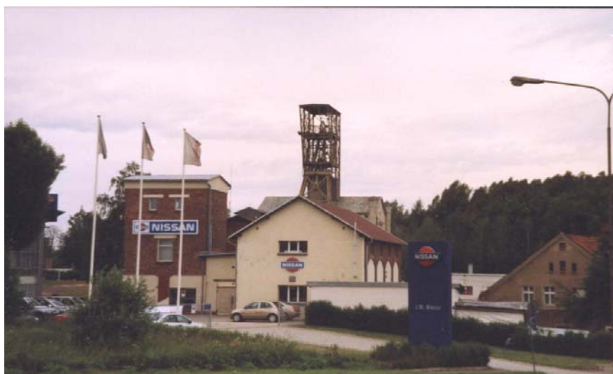
Fig. 1. General view of the adapted post-mine objects at the “Teresa” shaft.
