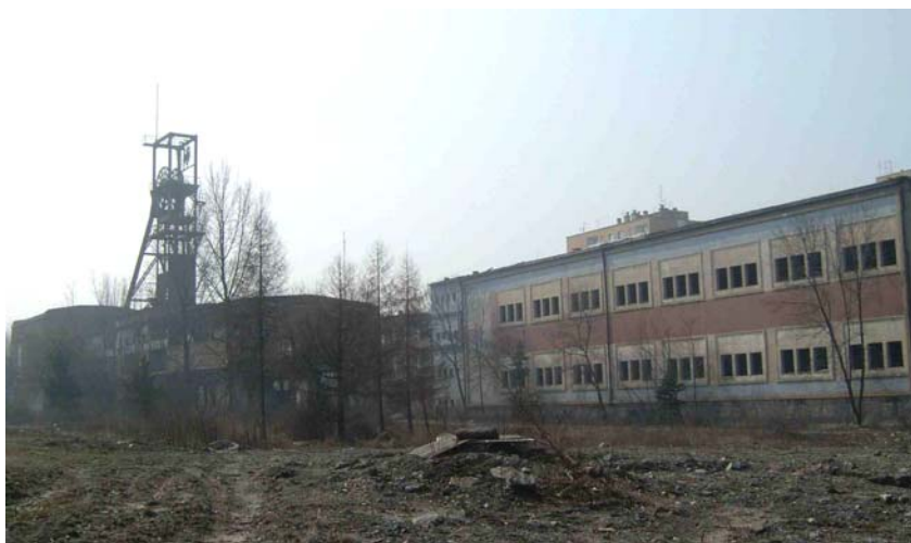
Fig. 4. Area of the former „Sosnowiec” mine – head gear of the „Anna” shaft with objects located close to the shaft and the administrative-social building
