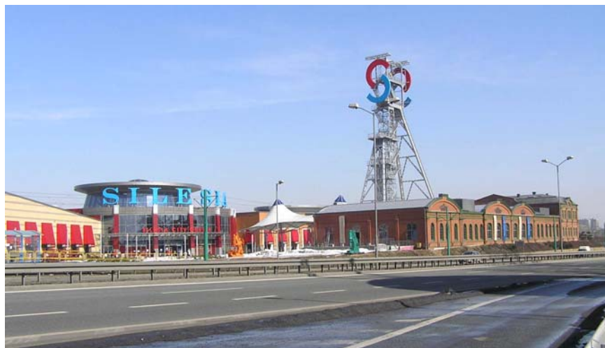
Fig. 7. General view of the Silesia City Center with the restored objects of the former „Gottwald” mine
