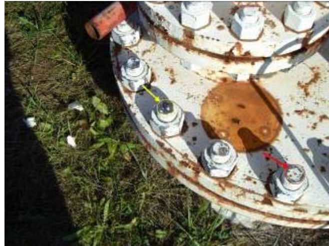
Fig. 1. Observed points stabilized upon reservoir neck.
