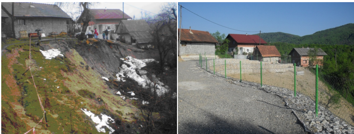
Fig. 7. Example of restoration solution for the landslide:
