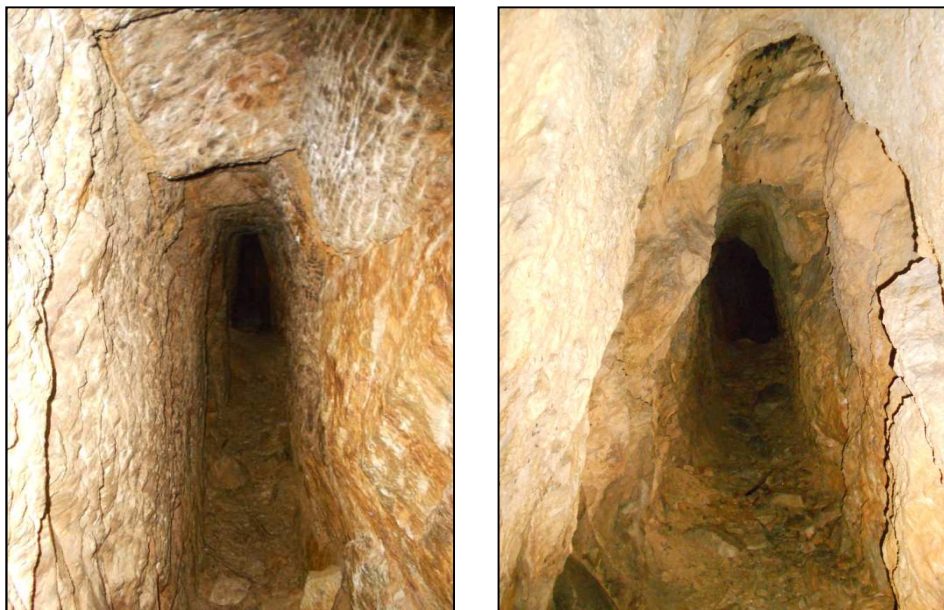
Fig. 8. Manually excavated medieval mining tunnels („kresanica“) by hammer and pick technology in the mining region Lubietová, locality Podlipa. Adit Upper Johan (left) and adit Uppermost Johan (right), (photo P. Hronček).
