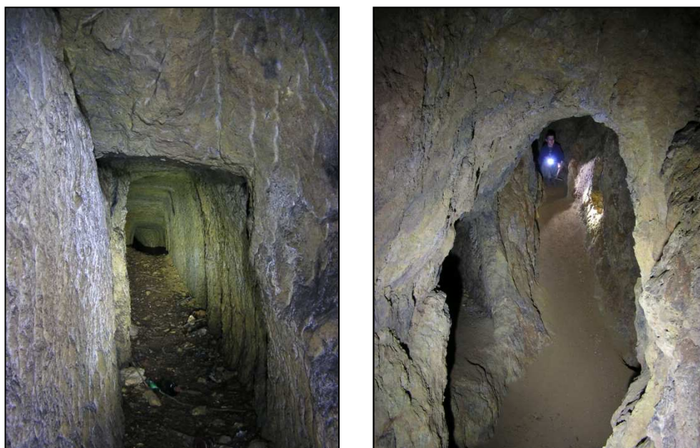
Fig. 9. Manually excavated medieval mining corridor („kresanica“) by a hammer and pick in the mining region Brezno, locality Skalka, excavated in dolomite (left). Underground spaces after manually mined of limonit deposit at locality Skalka (right) (photo V. Paprčka).
