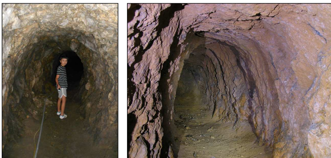
Fig. 17. Underground spaces created with black blasting powder (photo P. Hronček). Left: underground corridor under Lupča castle, dolomites (18th century). (Body height - 145 cm). Right: Name-less adit, location Skalka near Brezno, dolomites (half of the 20th century).
