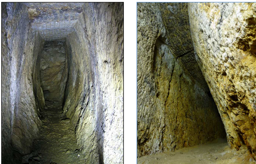
Fig. 13. Medieval adit Darius, Rožňava, probably excavated using fire disconnection and subsequently hammer and pick a technology (left), (photo V. Paprčka).
