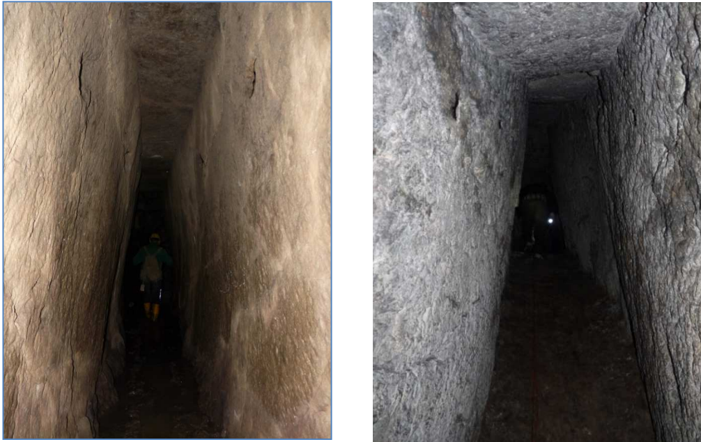
Fig. 10. Manually - by a hammer and pick excavated medieval mining tunnels („kresanica“) in Hodruša (district Žarnovica). Upper adit Ján (left) and Mine Starovšechsvätých (right). Relics after the ventilation space on both sides of the tunnels near ceiling. (photo K. Weis)
