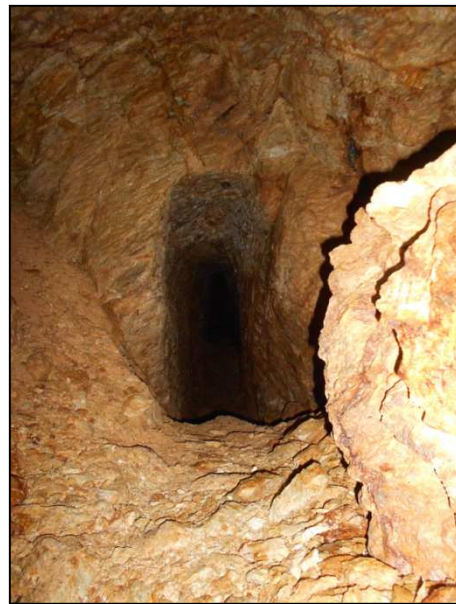
Fig. 7. Manually excavated mediaeval mining tunnels („kresanica“) by hammer and pick technology in the mining region Lubietová, locality Podlipa. Adit Lowest Johan (left) and adit Middle Johan (right), (photo P. Hronček).
