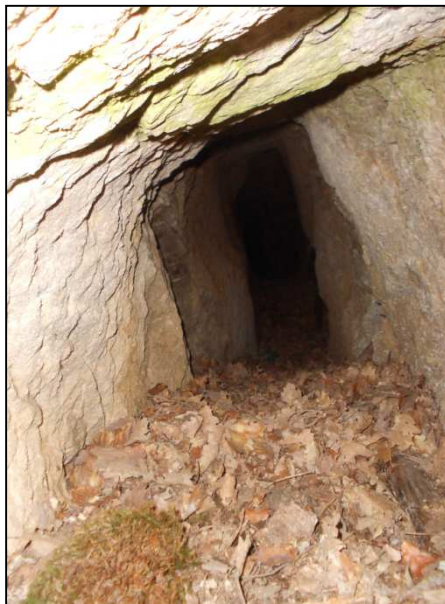
Fig. 7. Manually excavated mediaeval mining tunnels („kresanica“) by hammer and pick technology in the mining region Lubietová, locality Podlipa. Adit Lowest Johan (left) and adit Middle Johan (right), (photo P. Hronček).
