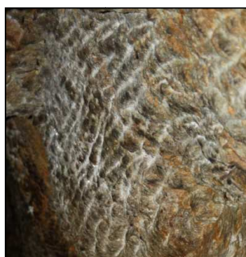
Fig. 4. Details of relics by manually disconnecting with hammer and pick. Adit Upper Johan in the mining region Lubietová, locality Podlipa. The nicks on the wall are cca 1,5 cm wide, cca 40 – 50 cm long and cca 0,5 – 1 cm deep. The distance ranges of nicks are 3-5 cm (left), (photo P. Hronček). Hodruša (district Žarnovica) - medieval mining Starovšechsvätých. Mining symbol – hammer and pick with Latin wrote the year 1510, manually disconnecting with a hammer and pick (right), (photo K. Weis).
