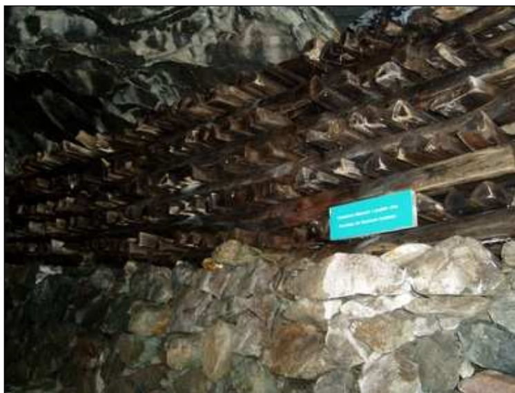
Fig. 12. The exposure of firesetting in Slovak Mining Museum Banská Štiavnica (photo P. Hronček).
