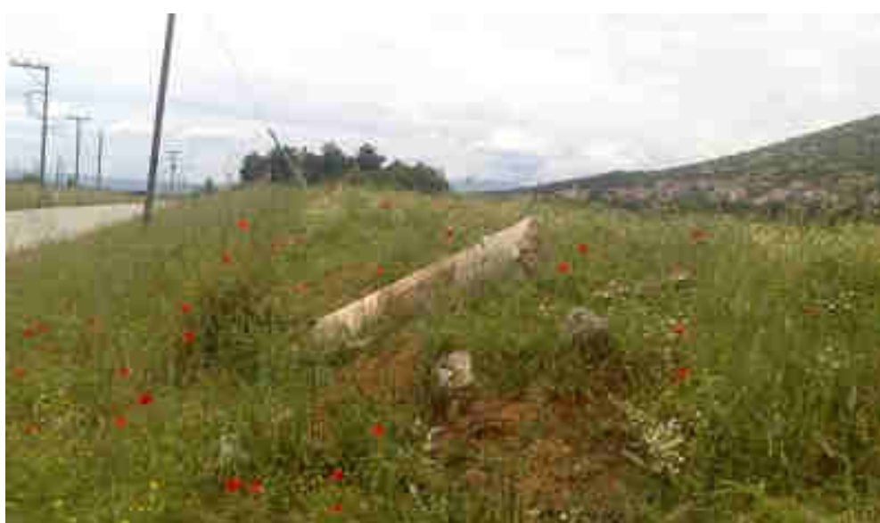
Fig. 4. Control Point 96069 (destroyed).
