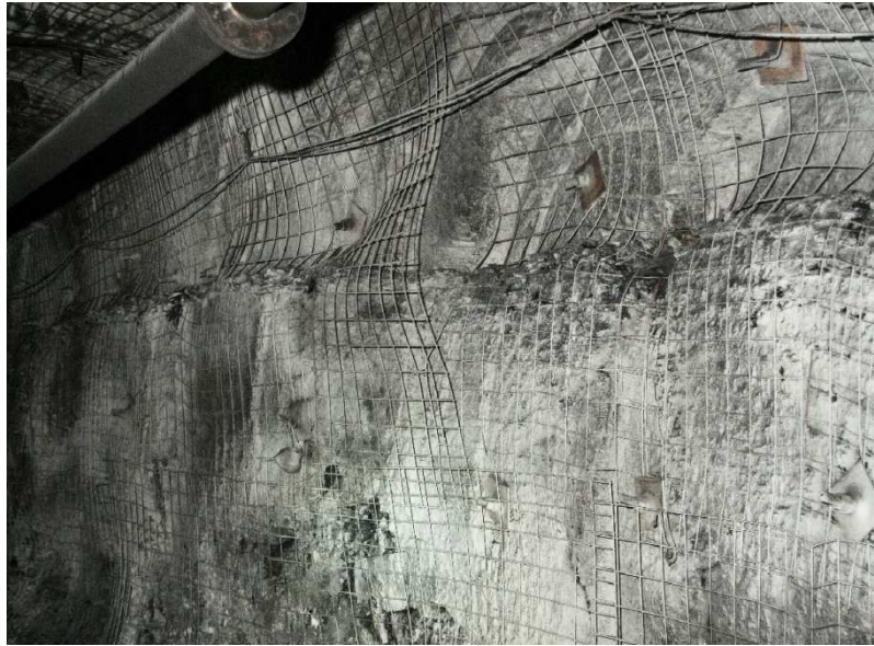
Fig. 4. Documentation on bolting road walls.
