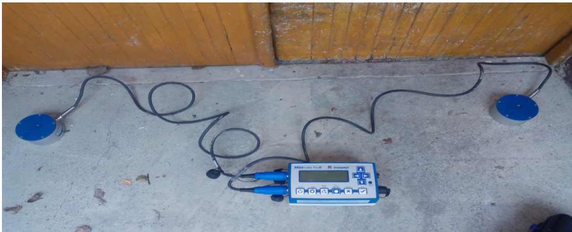
Fig. 13. Location of MINIMATE PRO 6 on the foundations of a residential building (Fehér et al., 2019)
