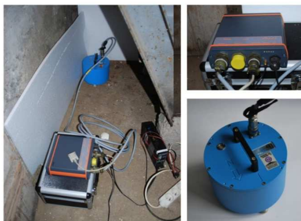
Fig. 2. Apparatus GAIA Q with seismometer Lennartz LE-3D/5s is installed in the cellar of a small masonry building at a depth of approximately 2 meters below the surface.
