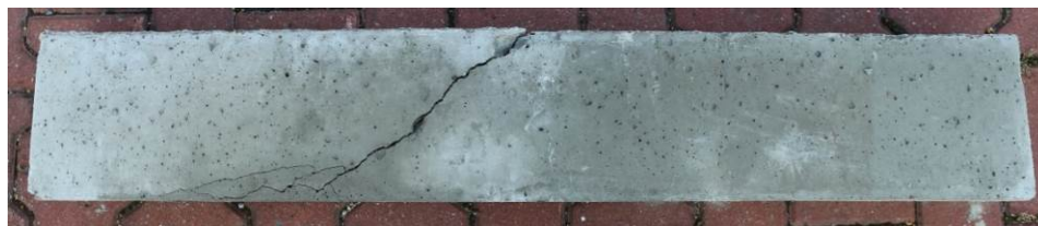
Fig. 17. Beam after the test – shear crack
