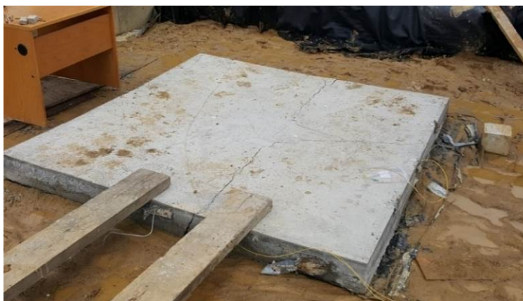
Fig. 26. Concrete slab with crack - after the test
