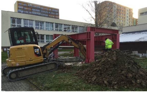
Fig. 5. Subsoil replacement
