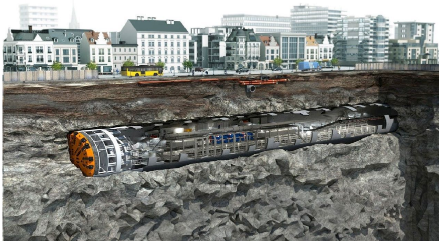
Fig. 3. Construction of a metro tunnel with a TBM
