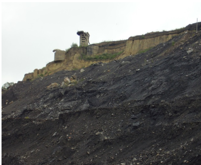
Fig. 1. The safety pillar under the industrial site of the Northern Maganak mine, Kuzbass
