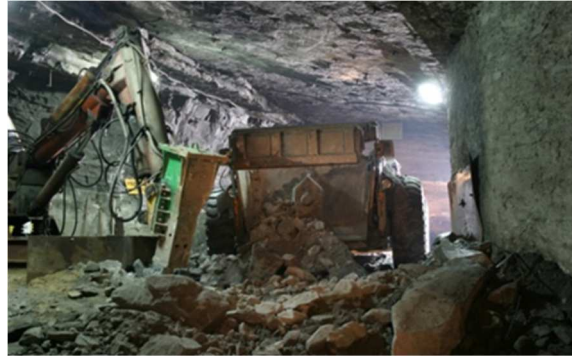
Fig. 7. Unloading the haul truck on the grate
