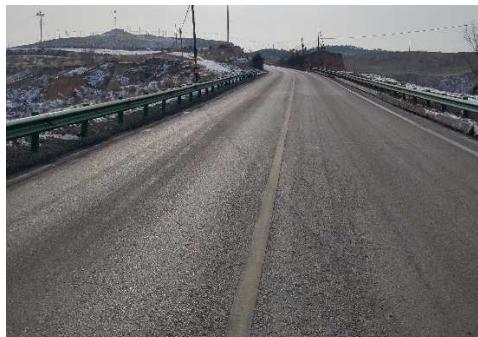
Fig. 11. Opening to traffic conditions of the testing section
