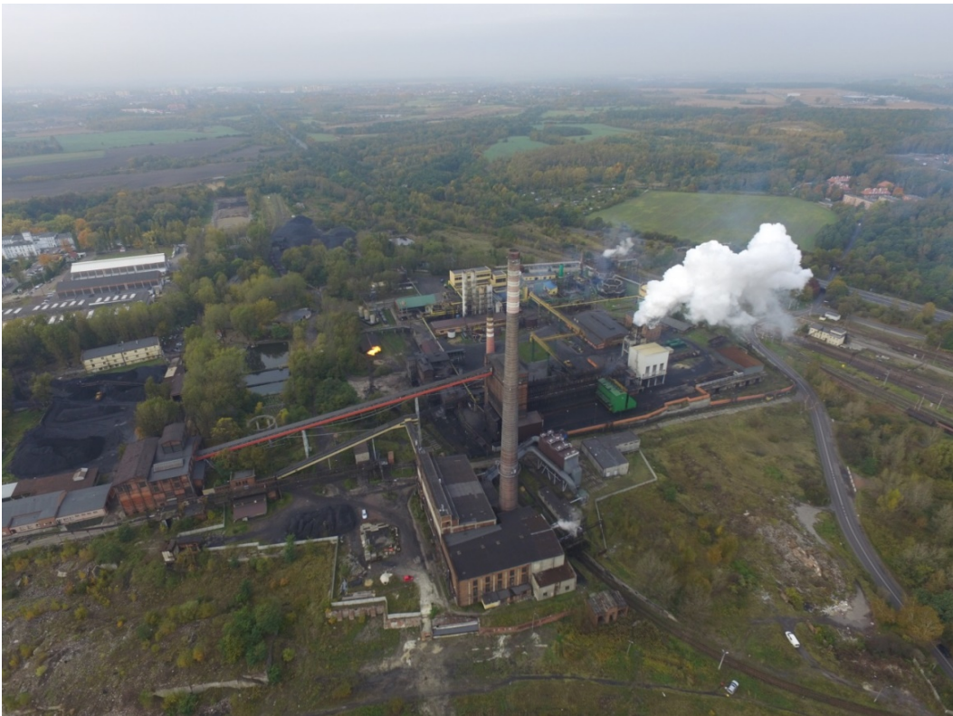
Figure 1. Coking plant and high chimney under which partial operation was carried out
