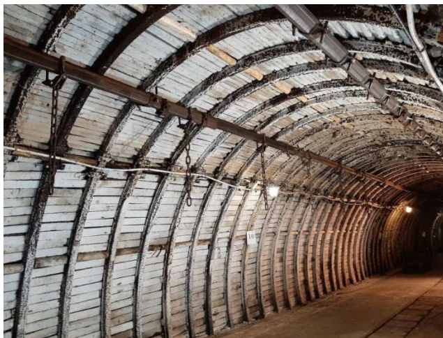
Fig. 20. Space prepared for in-situ testing
