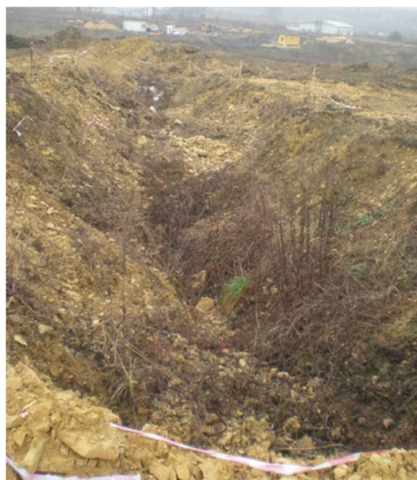
Fig. 2. A sinkhole caused by shallow mining of zinc and lead ore in the area of the A1 motorway construction site, Poland
