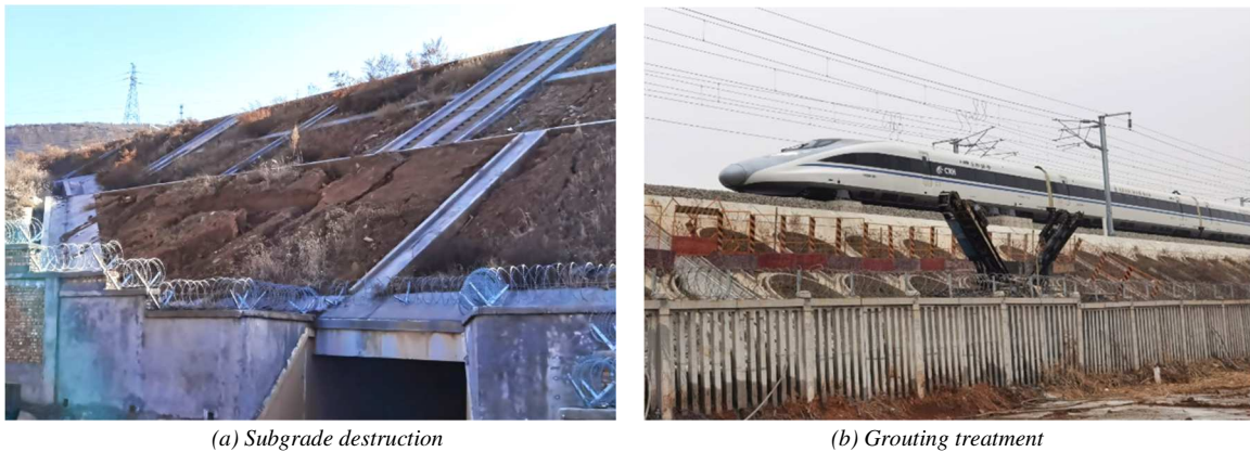
Fig. 1. Damage and treatment of the subgrade after the heavy rainfall.
