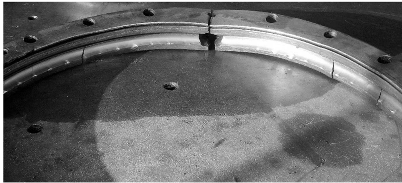
Fig. 6. Damage to large parts of the raceway and fractures of the bearing ring
