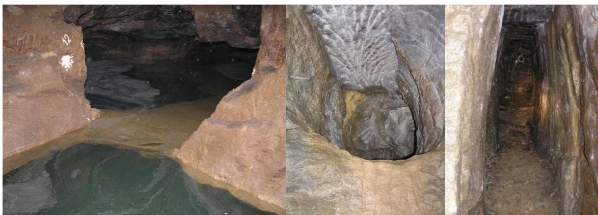
Fig. 6 Photos taken in the historical parts of the mine (fire setting, extraction using a picker and miner's hammer, underhand stopping or overhand stopping); photo: Lednická
