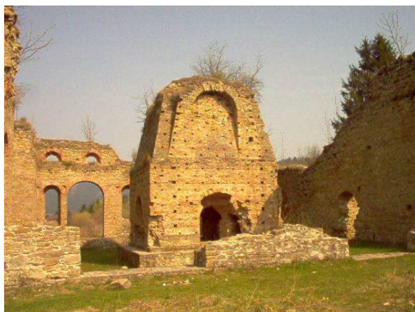
Fig. 5. The blast furnace in Podbiel.
