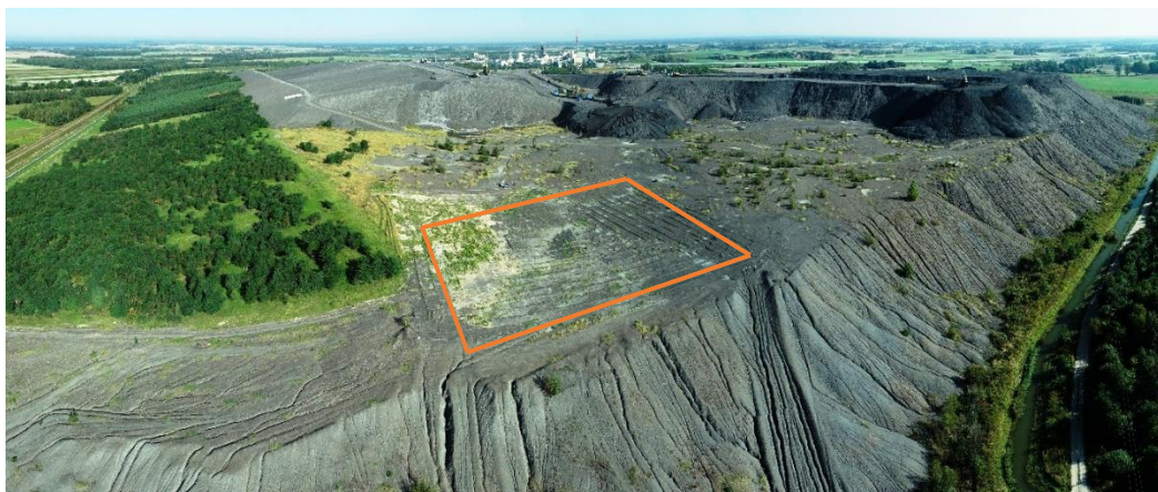
Figure 1 LW "Bogdanka" Mine Waste Neutralization Facility – under construction, partially recultivated slopes
