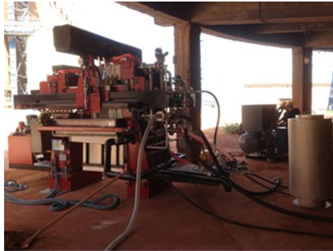
Fig. 4. Pilot sized press filter installed in the red sludge washing circuit.
