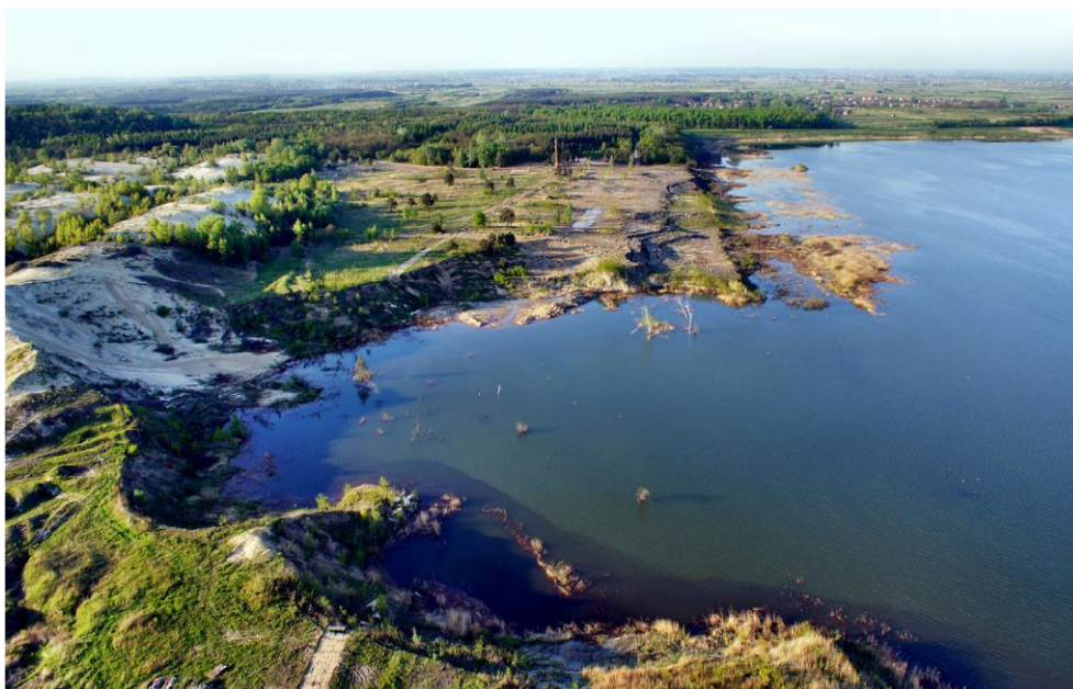
Fig. 9. Fragment of the reservoir, visible effects of land slide disaster Source: (Biernat G. www.parafoto.pl )
