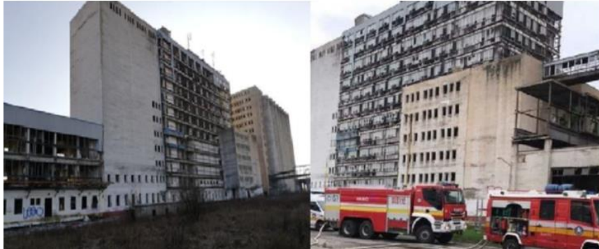
Fig. 7. The building where the fire took place (source: elaborated by authors)
