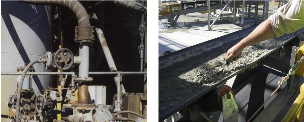
Fig.1 Manual and automatic sampling in the plant.
